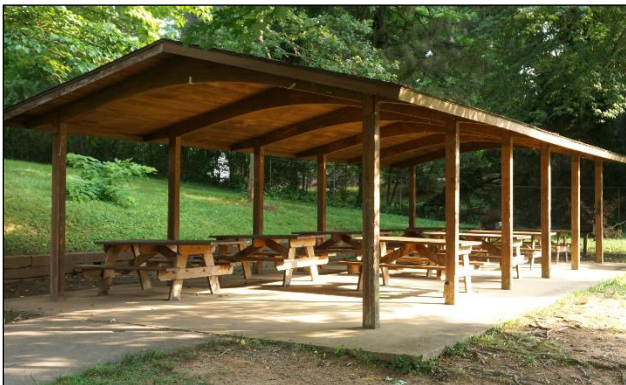
Picnic Shelter at Murphy-Oakley Park
